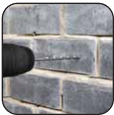
SDS Drill for drilling pilot hole
