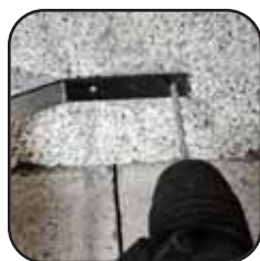
Spacing template for cutting double back box holes
