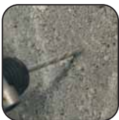
SDS Drill for drilling pilot hole
